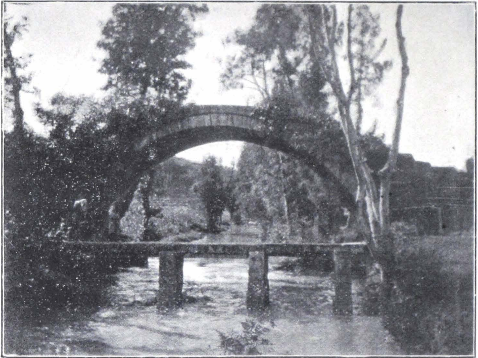
A high arched and stone Slab bridge in conjunction, The latter is at road level.
